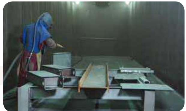
Pneumatic blasting chamber
